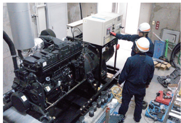
Test Run for Emergency Generator Replacement Project
